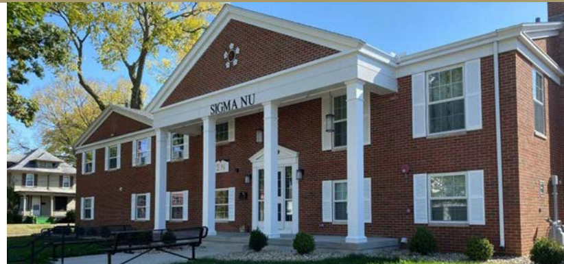
Completed Phase II renovations on the front of the chapter house.
